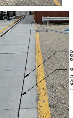
CONTRACTOR TO PROTECT EXISTING SIDEWALK. PLACE EXPANSION BETWEEN SIDEWALK AND NEW PARKING LOT
