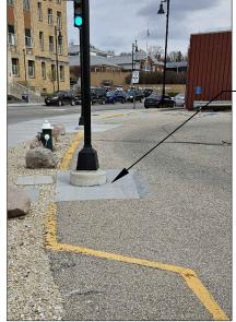
CONTRACTOR TO PROTECT EXISTING LIGHT POLES AND DOWEL INTO EXISTING CONCRETE
